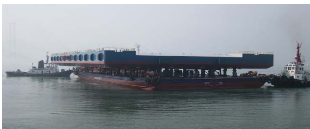
▲ Seaborne transport of the pontoon (waiting for entry into the Gwangyang container facility)
