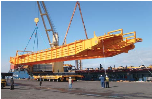
▲ Ready for ship loading - Bucket Wheel Boom
