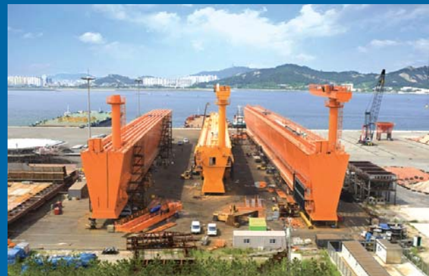
▲ Port P.E. operation
