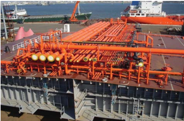
▲ Secondary UNIT installation after P,E.
