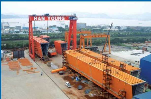
▲ Factory P.E. operation
