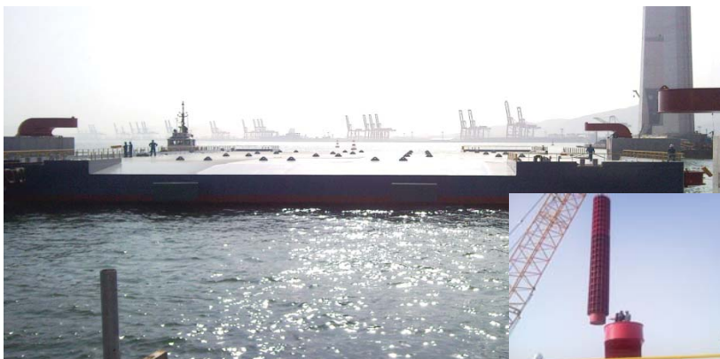
▲ Pontoon installation and top device installation
