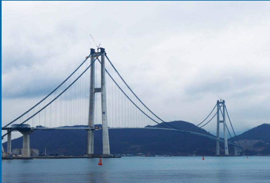
▲ View of the Yi Sun-Sin suspension bridge site
