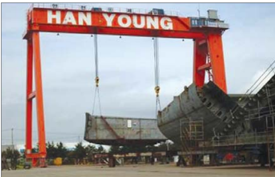
▶ Gantry crane 320tons
