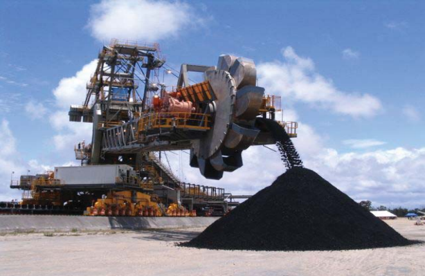
▲ Picture of trial running on site
