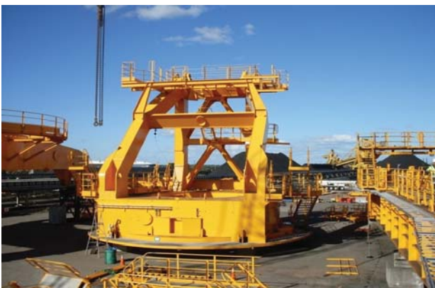
▲ Picture of trial running on site
