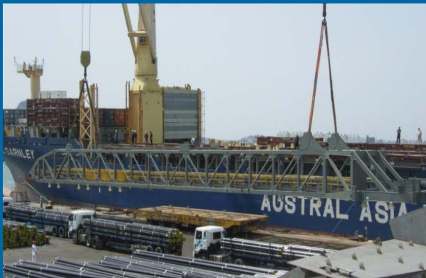
▲ Ship loading : B/W BOOM (Weight : About 120ton)
