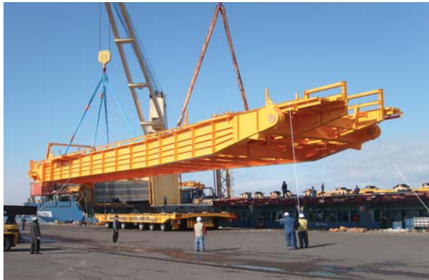
▲ Ready for ship loading - Bucket Wheel Boom
