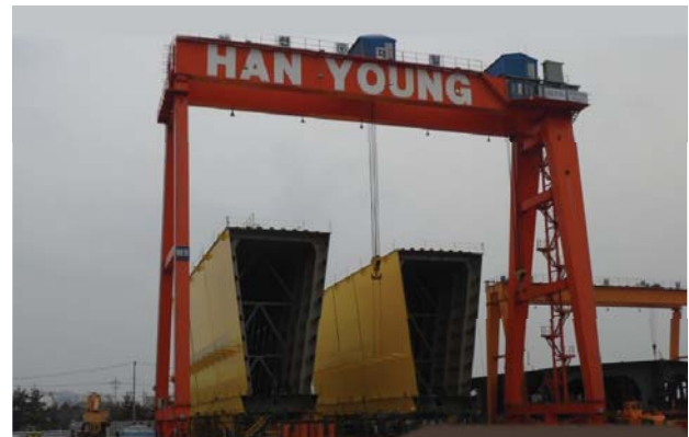
▲ GIRDER (UPPER + LOWER) P.E
